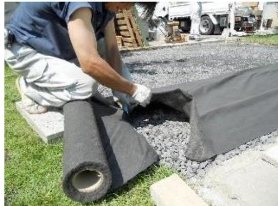
5. Spread low fines bedding material to a uniform depth over unwovengeotextile, working no more than 1-2 metres ahead of laid paving units.
