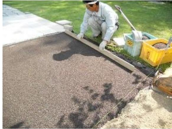
8. Immediately after screeding, lay main body of area with 60 mm thick Cerama Pave permeable pavers. Use a mechanical device to cleanly cut pavers. Adjust surface levels of laid pavers with rubber hammer.
