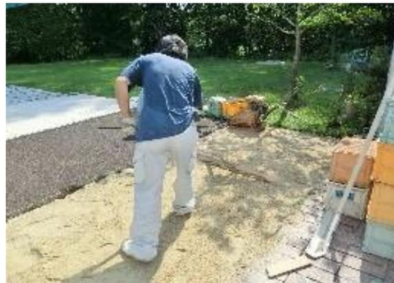
6. Compact to depth of 30 mm: 3-5 passes at 30-40 metres per minute using a plate compactor having a minimum plate area of  $0.25 \text{ m}^2$ ; minimum effective force per unit of plate of  $75 \text{ kN/m}^2$ ; frequency of 65-100 Hz; and minimum mass of 200 kg.
