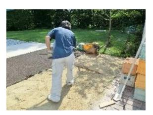
6. Compact to depth of 30 mm: 3-5 passes at 30-40 metres per minute using a plate compactor having a minimum plate area of 0.25  $\text{m}^2$ ; minimum effective force per unit of plate of 75 kN/m<sup>2</sup>; frequency of 65-100 Hz; and minimum mass of 200 kg.
