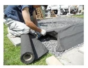
5. Spread low fines bedding material to a uniform depth over unwovengeotextile, working no more than 1-2 metres ahead of laid paving units.
