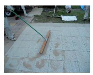
11. Compact pavement with rubber plated compactor: 3-5 times at 30-40 metres per minute. Add joint filler as required to fully fill joints then compact again.
