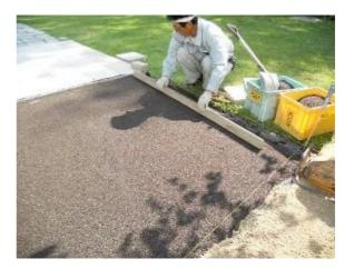
8. Immediately after screeding, lay main body of area with 60 mm thick Cerama Pave permeable pavers. Use a mechanical device to cleanly cut pavers. Adjust surface levels of laid pavers with rubber hammer.
